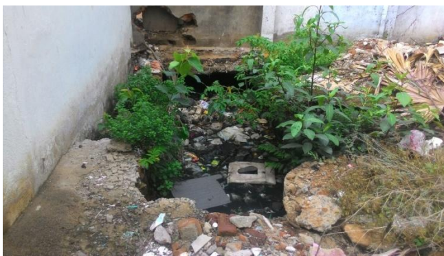
Condition of Storm water drain on 2nd main road
