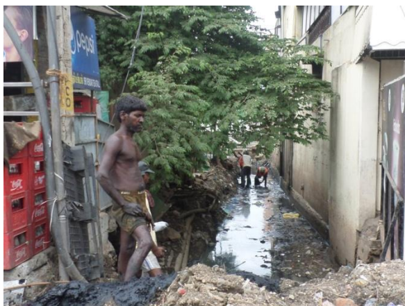
GST Road canal near police station
