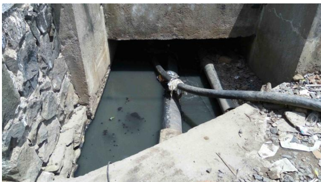
Culvert under the railway track
