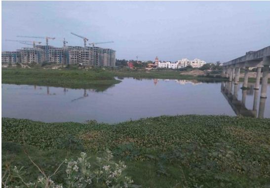
After 2.4 Kms, the bund in between remains
