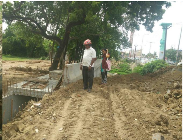
Canal being closed down with sand near MGR house
