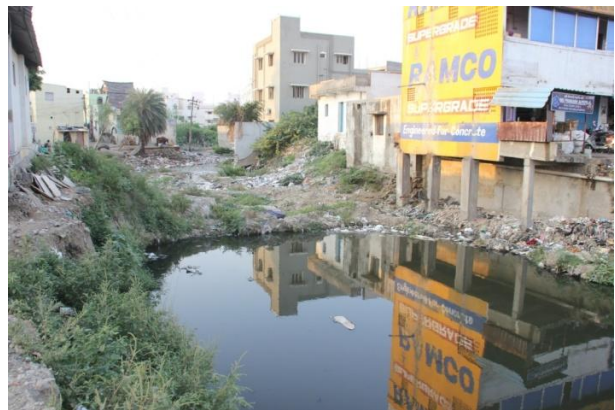
Encroachment on right and flow in the middle blocked by garbage and debris
