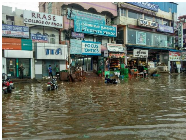
GST Road during floods near Chrompet police station
